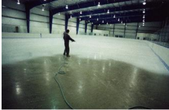
Fig. 15. Making the ice sheet in an ice rink.
